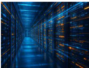
Generative AI 2025 - Computing and AI for Data Center
